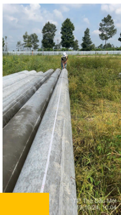
Inspection of the piles
